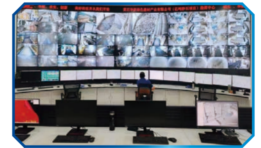
Intelligent hundred million-ton sand plant (Central Control Room)
