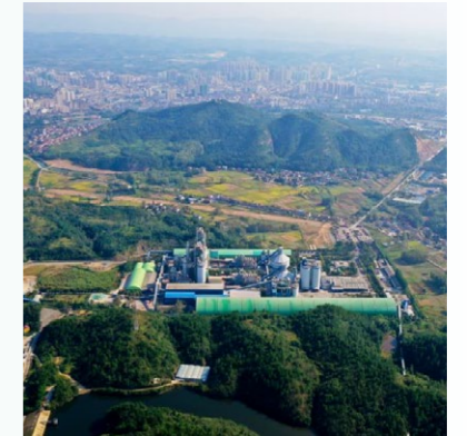
The "Beautiful Factory" construction of Xiangyang Factory
