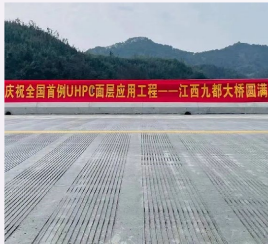
Chaokelong applied in the reconstruction of Jiudu Bridge in Shangrao's Dexing, Jiangxi Province
