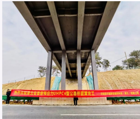
Chaokelong applied in the fully prefabricated UHPC flyover of Macheng-Ankang Expressway
